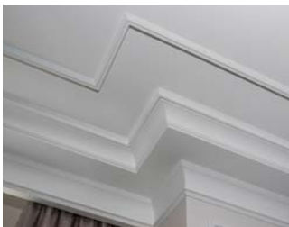
CABINETS, TRIM & CROWN MOLDING
